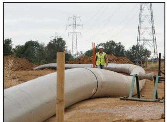
GPS was awarded the order for the supply of 710mm diameter Excel (PE100) pipe. The pipe was supplied in SDR 21, which denotes the wall thickness. By careful investigation of the actual pressure and capacity requirements, substantial project savings were made by using the SDR 21 specification, rather
